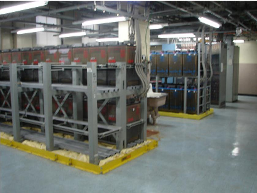
**Figure 2. The -48V VLA battery strings are approximately 190 KWh each.**
