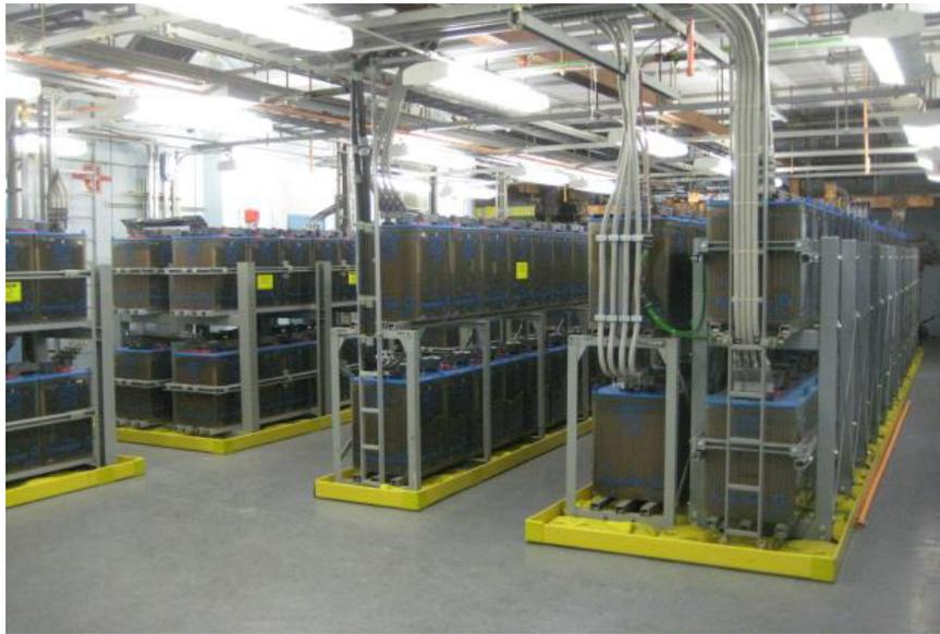
**Figure 4. Battery room with more than 1400 KWh capacity. For these lead-acid batteries, it is allowable (unlimited), but other technologies have 200 KWh or 600 KWh limits before the facility is regulated as high hazard occupancy.**
