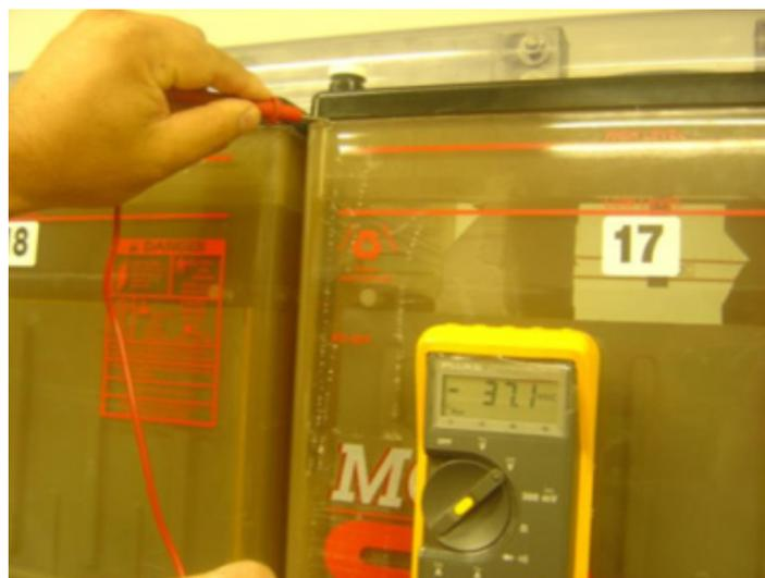
**Figure 7. A leaking container-to-cover seal could result in a battery fire.**
