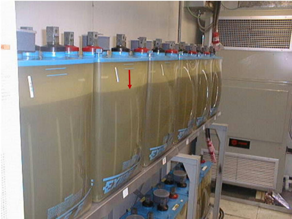
**Figure 5. Lead calcium battery cells with containers that bulged due to an overheat condition in the wake of an HVAC system failure. Note the drastic electrolyte level drop (Arrows) that resulted from container bulging.**
