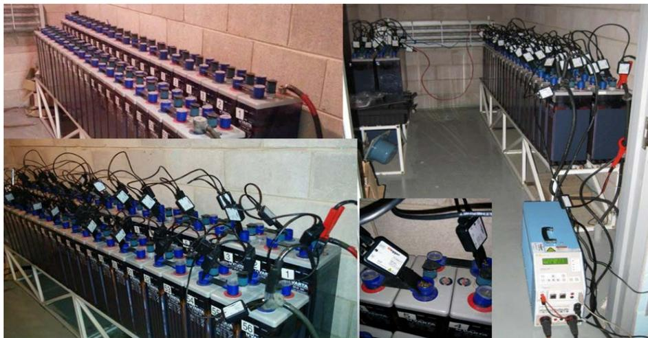
**Figure 2: Connection of BVM's and load bank to the battery**
