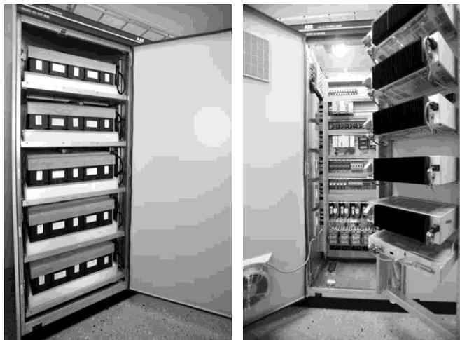
**Figure 1. The 5 battery strings are placed on individual sliding shelves (left), Battery chargers are placed on the back of the second cabinet door and the BMCs on the left hand side wall (right).**
