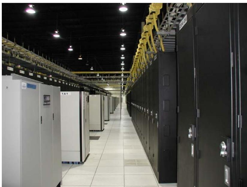
**Figure 4. Rows of UPS fed Power Distributing Units (gray cabinets) feeding power to rows of IT equipment (Black cabinets)**
