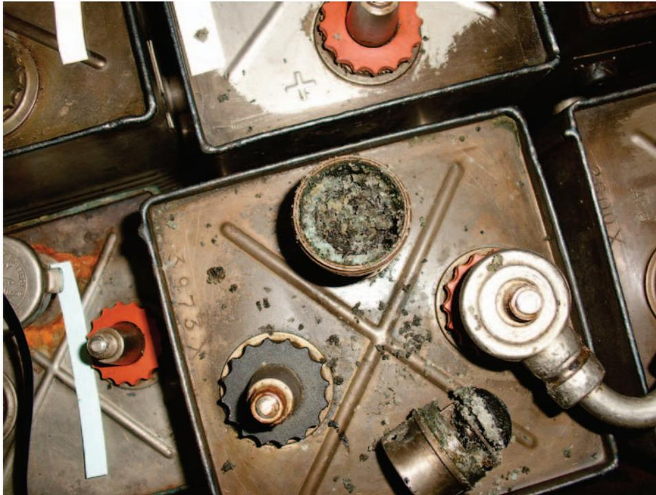
**Figure 3. The carbonate build up in one vent tube**
