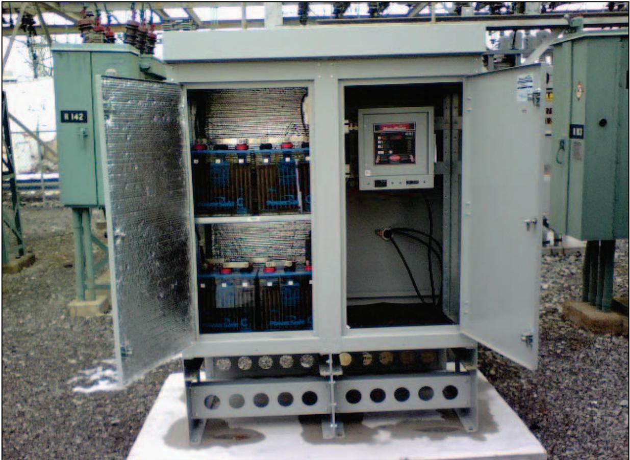
**Battery and battery charger used in a switchgear application.**
