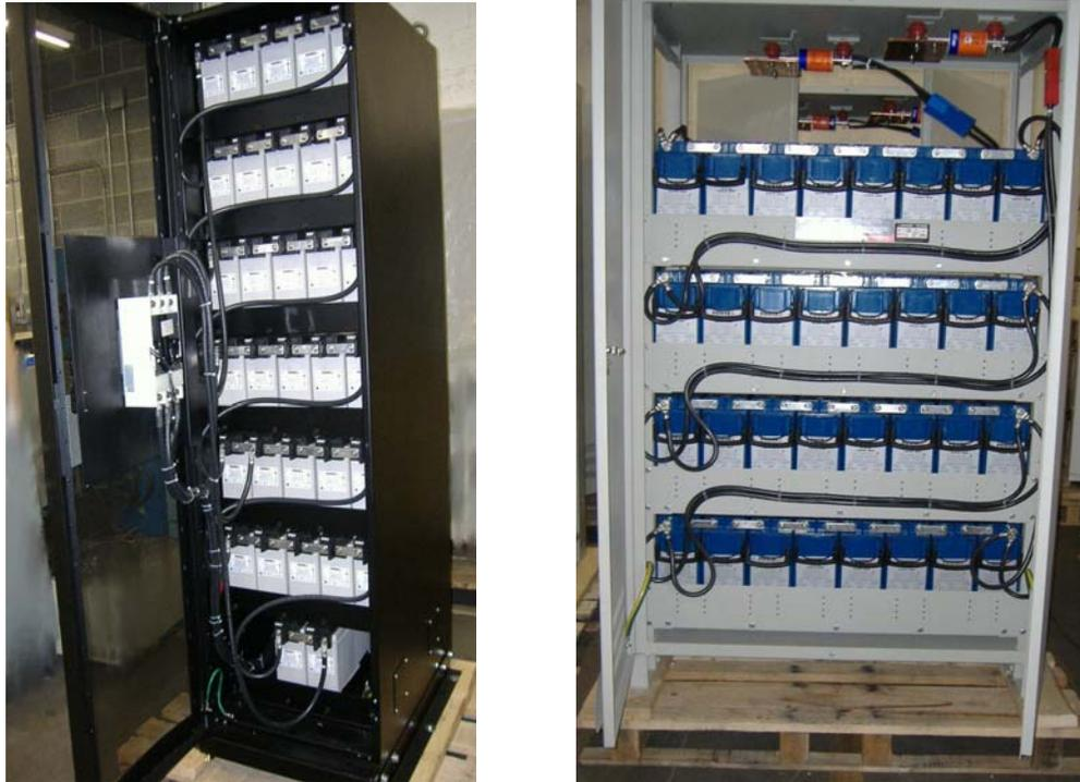
**Figure 3. Ten Year Front Access Batteries in Cabinets.**
