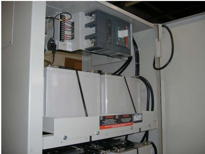
**Figure 2. Close-up of 10Yr. Top Terminal Battery Installed in Cabinet.**
