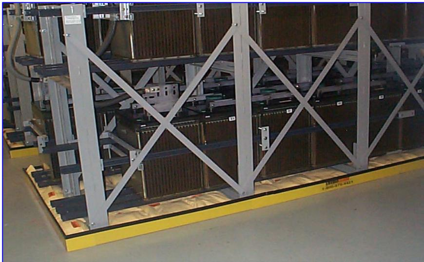
**Figure 4 – 4” Spill Containment System
